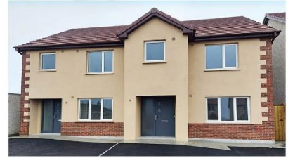
17 UNITS AT LIMEGROVE, FERRYBANK
