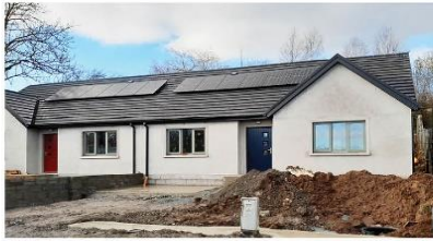
2 UNITS AT MULLINAVAT
